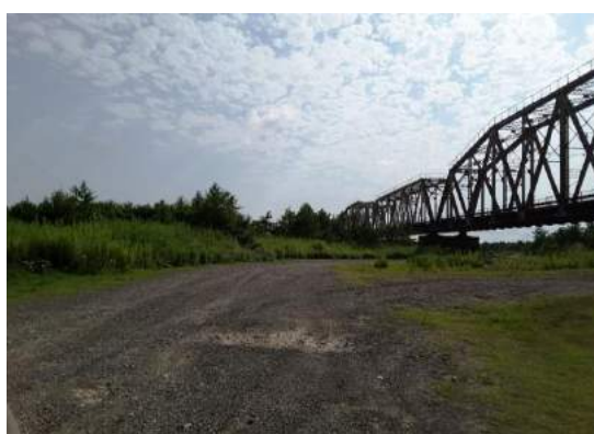
Vegetation near railroad bridge
