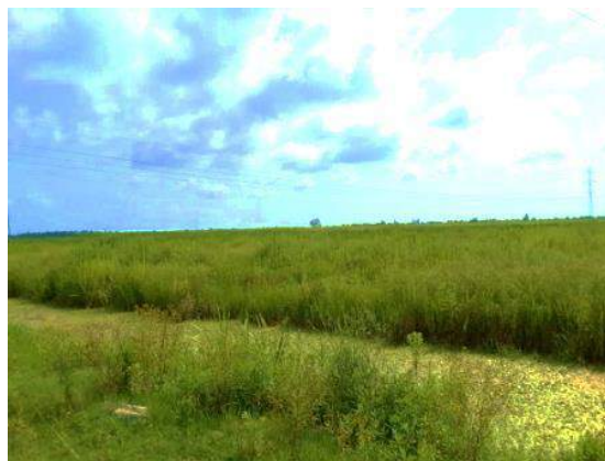
Drainage canal overgrown with amorpha
