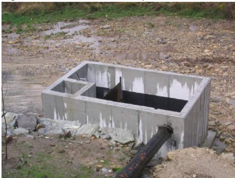
Figure 13. Retention Chamber: Operation Phase
